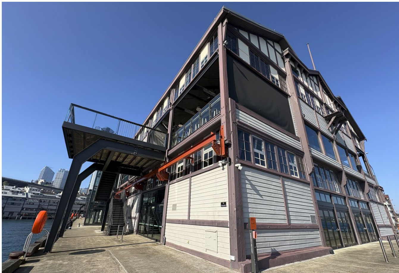
Contemporary additions on Piers 4/5
